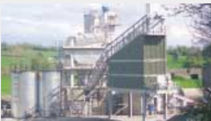
210 tonne mixed material storage
